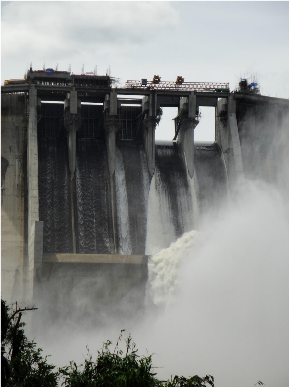
Sinohydro's Kamchay dam in Cambodia, financed by China Eximbank (Photo by Inclusive Development International)
