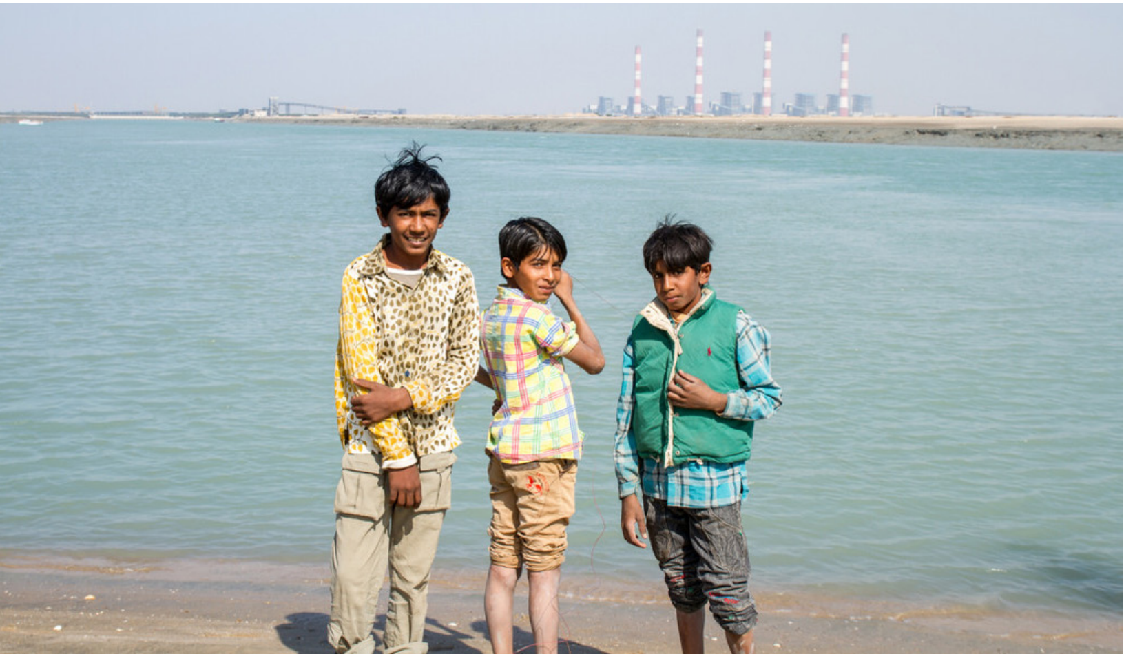
The Mundra complex, located in Gujarat state, includes a coal plant, port and special economic zone. It has polluted the ocean and displaced local fishing families. The IFC's commercial bank clients financed both the complex and the company that owns it, Adani. Photo © Joe Athialy
