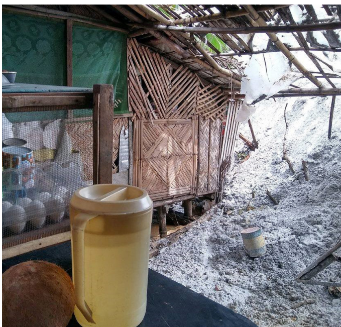
Coal ash seeps into a home in Bataan Province. The corporate bond market, through which companies raise capital to build coal plants, presents an accountability gap for the IFC and the wider financial system. Photo by Derek Cabe.
