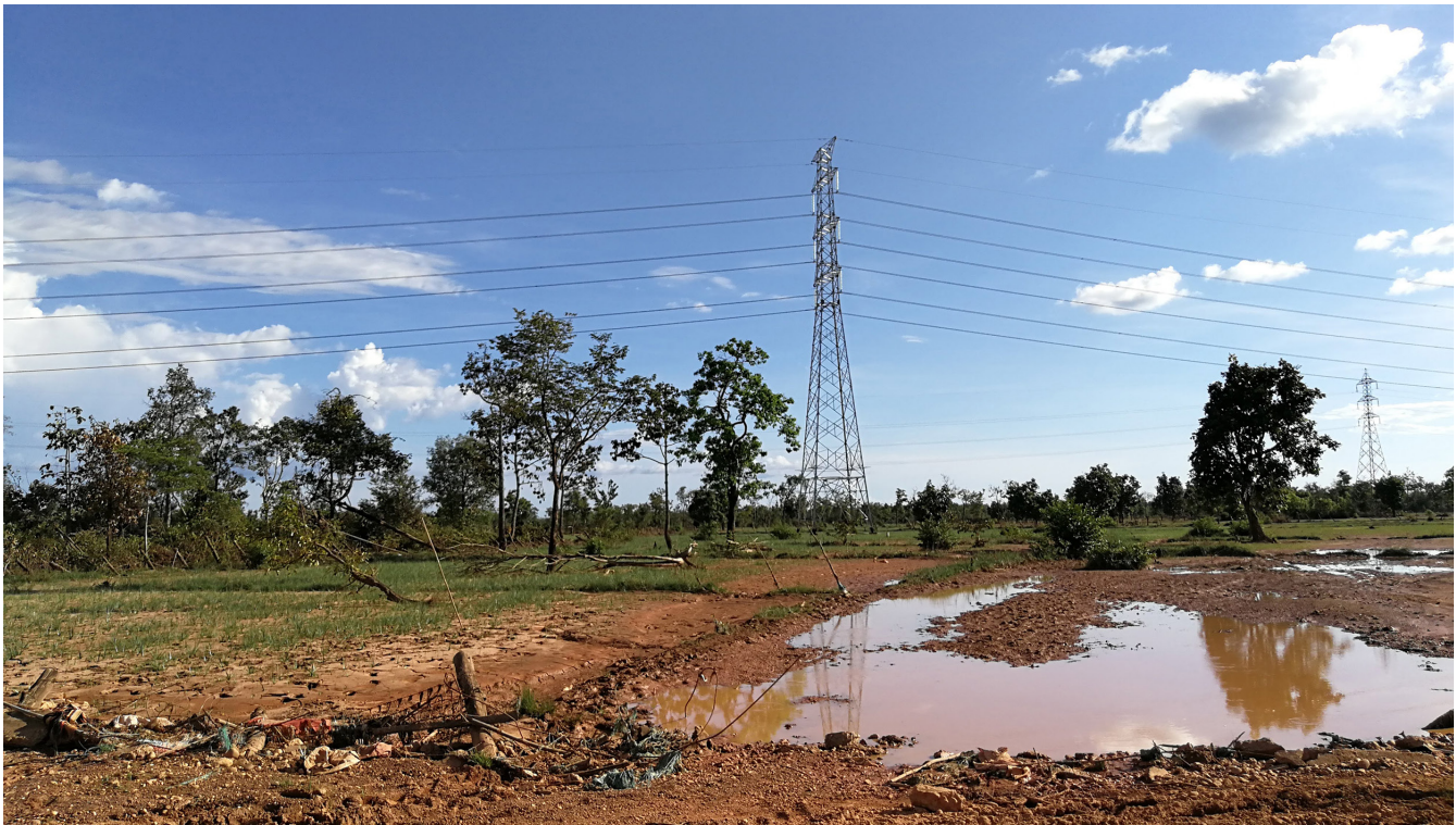
Dam collapse flood-affected area (Photo Credit International Rivers, October 2018)
