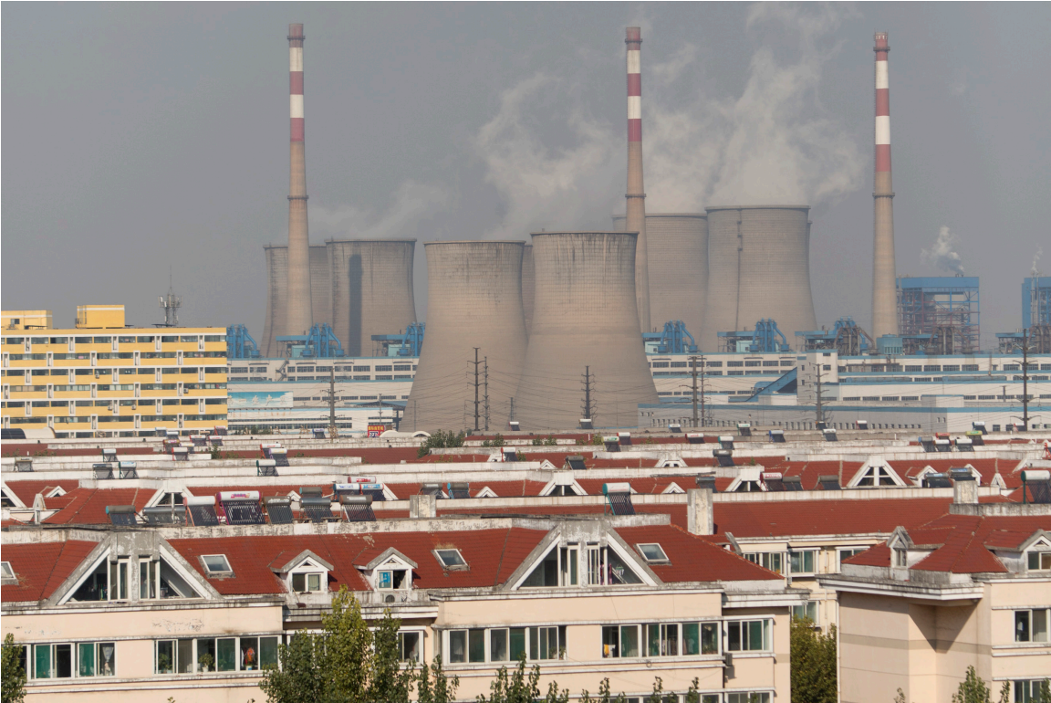
The cooling towers of a coal power plant at the China Hongqiao Group, Ltd. aluminum smelting facility in Zouping, China. Aluminum producers' reliance on coal means that each year the industry is responsible for about one billion tons of CO 2 equivalent or around two percent of global greenhouse gas emissions. © 2013 Brent Lewin/Bloomberg/Getty Images
