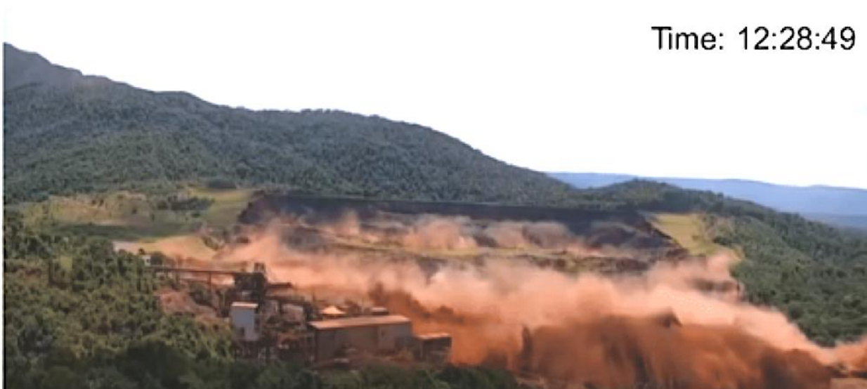
Figure 2 Brumindinho TSF failure 2018
