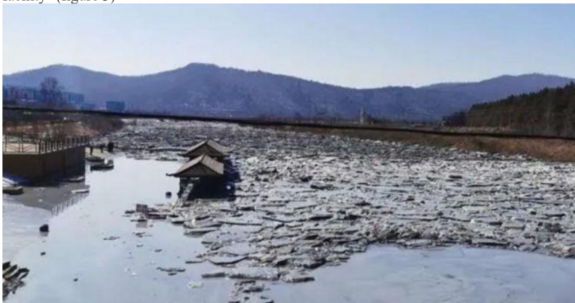
Figure 3 An unstable foundation may also lead to a TSF spill that would not necessarily destroy villages, but rather flood downstream streams with toxic waste as here last year at China's Yichun Luming TSF.
