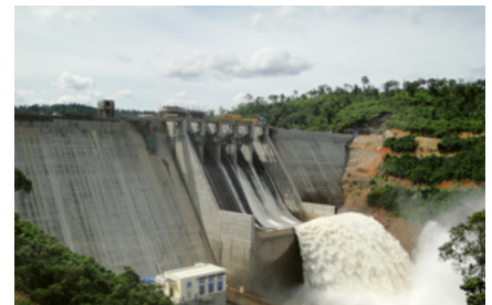
ABOVE: SINOHYDRO'S KAMCHAY DAM, CAMBODIA.
