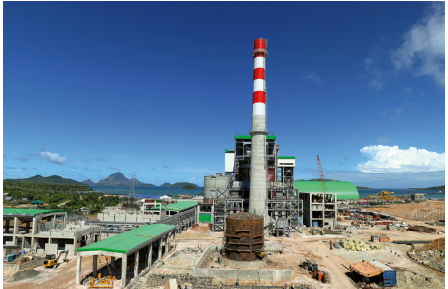
ABOVE: CONSTRUCTION OF A COAL FIRED POWER PLANT IN THE PHILIPPINES.
