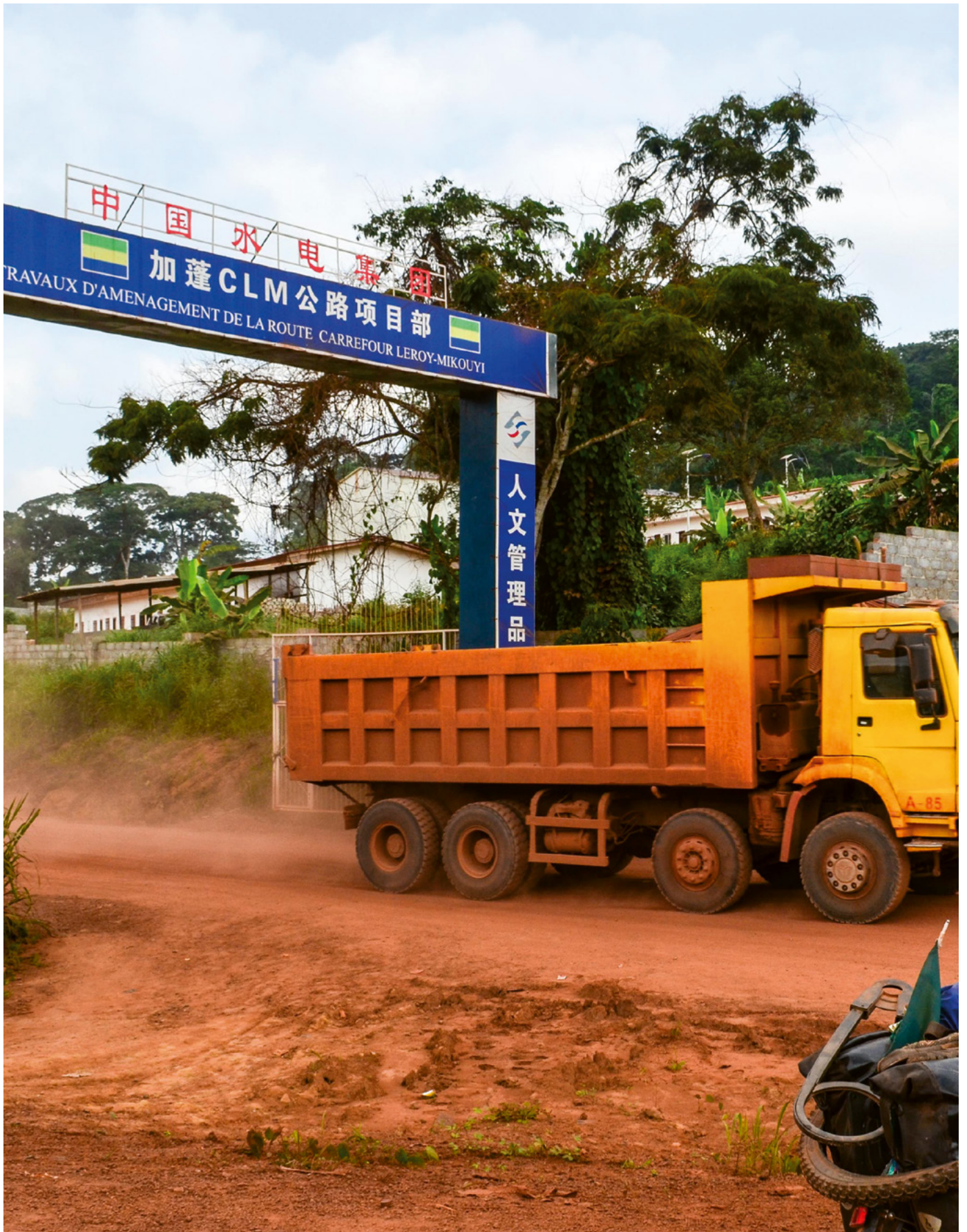
ABOVE: ROAD CONSTRUCTION FOR CHINA'S SINOHYDRO IN GABON.
